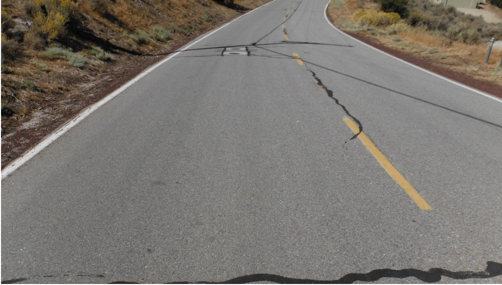
Jacaranda Drive, Section 08, PCI = 83
