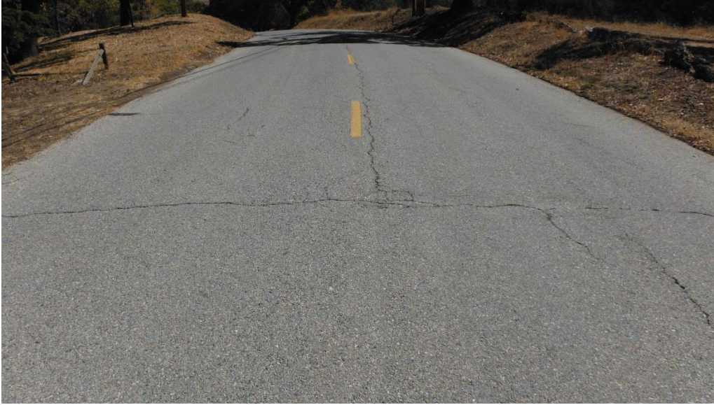
Pinedale Drive, Section 04, PCI = 63
